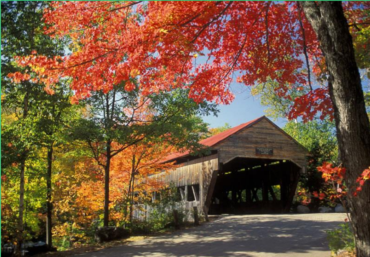
Albany Covered Bridge
